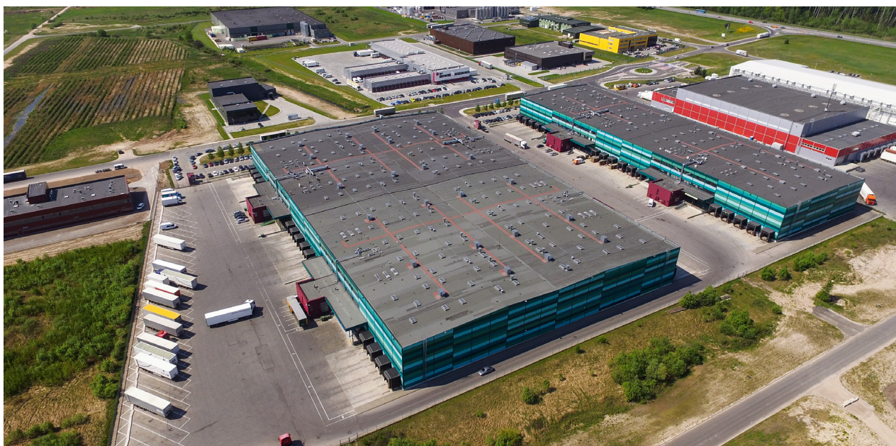
Kaunas Terminal logistics centre in Lithuania
